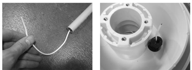
4. Thread a thin piece of cord or tough string through the cable conduit from the beginning of the conduit (near the transformer) all the way through to the light niche. This will be used to pull the light's power cable through later on. We recommend using sweeping bends and not elbows, to make it easier to pull the cable through.
