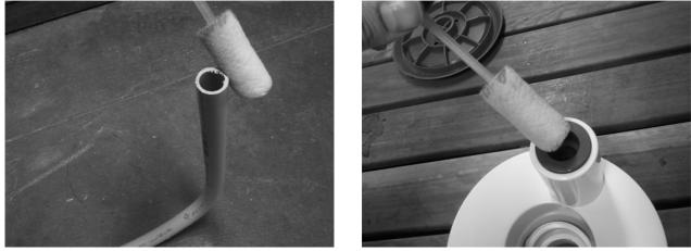
5. Apply PVC solvent primer to the conduit adaptor and to the conduit. Allow to rest for one minute, then apply PVC solvent cement (non-pressure type N is sufficient) to both parts.
