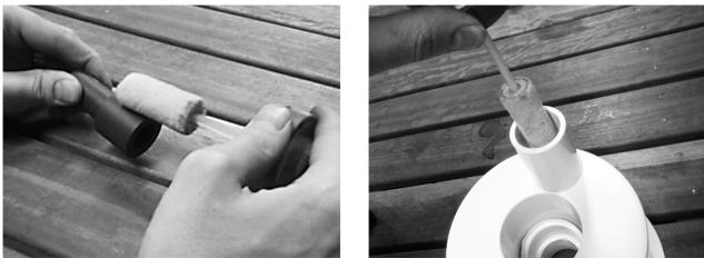
1. Apply PVC solvent primer to the conduit adaptor and to the socket on the niche. Allow to rest for one minute, then apply PVC solvent cement (non-pressure type N is sufficient) to both parts.
