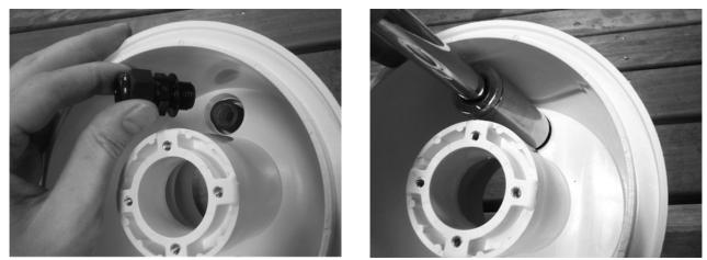
3. Insert the cable gland into the threaded socket on the conduit adaptor, ensure the rubber washer is on the thread of the cable gland. Tighten with a socket wrench.
